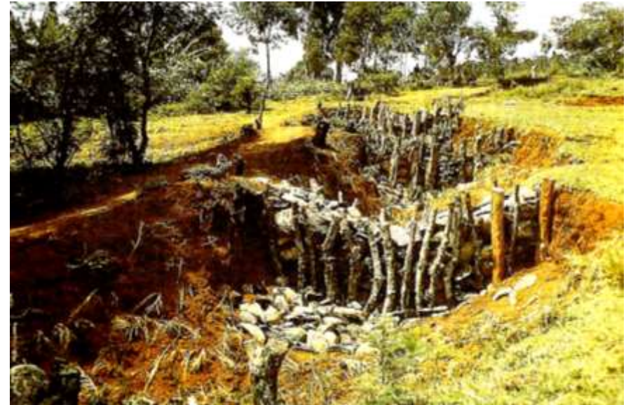
Check dam to control gully erosion
